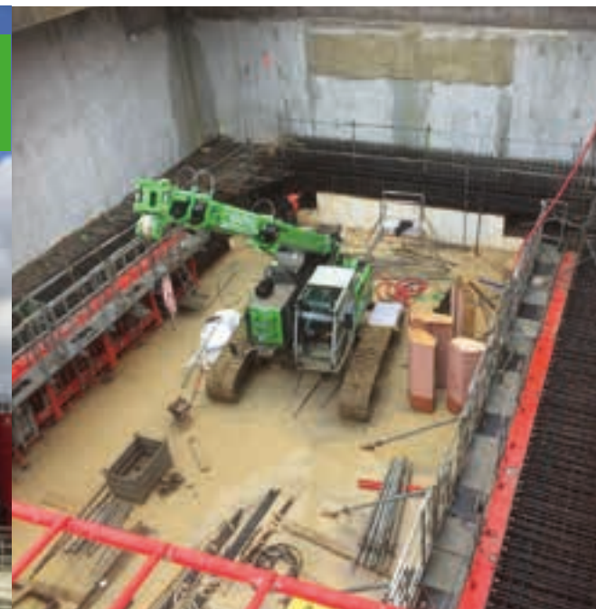
A SENNEBOGEN 6113 E as service crane.
